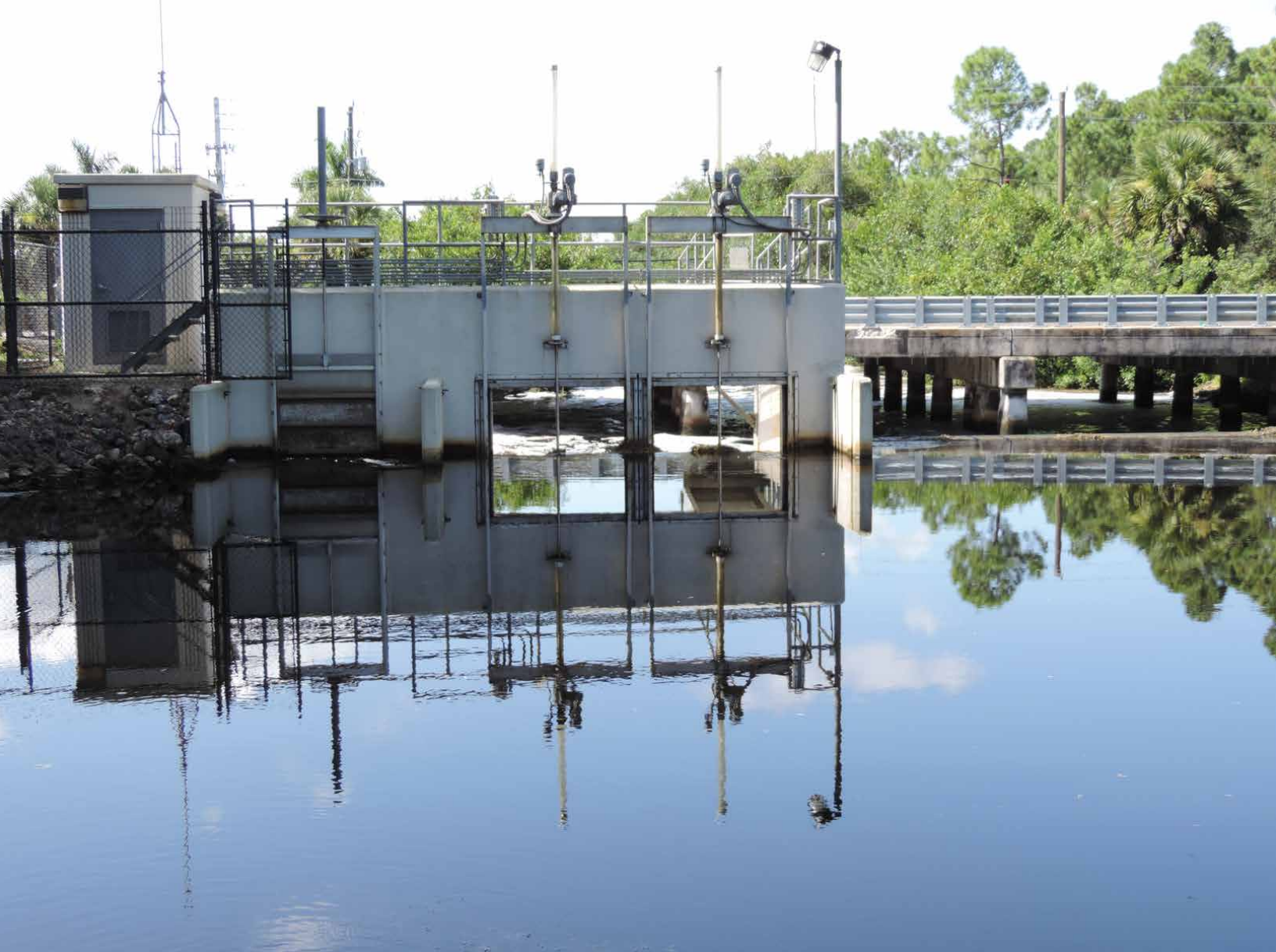
Current water management on Henderson Creek includes the opening and closing of a weir to control water flow.
